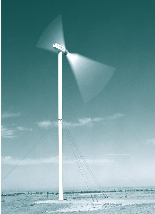
This 500-kilowatt engineering and manufacturing development wind turbine, of the sort encouraged by new California laws, is installed at the Fairmont Reservoir of the Los Angeles Department of Water and Power. The turbine is grid-connected and features a downwind rotor, hinged blades that flex, and soft towers that bend slightly to reduce loads on the other components.
